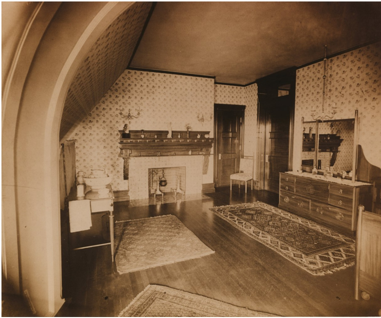
Southwest Tower Room
